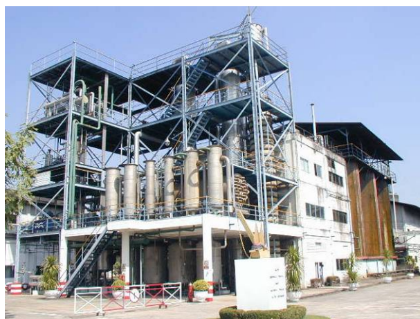
Fig. 6.5.2. Ethanol production plant in Thailand.
