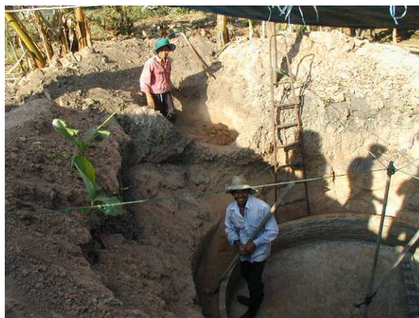
Fig. 6.5.1. Fermentation reactor under construction.
