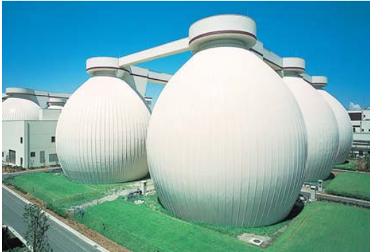
Fig. 8.2.2. Example of a large scale sewage sludge anaerobic digester. (Northern second sewage treatment plant)
