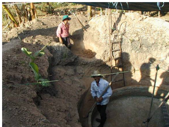
Fig. 6.5.1. Fermentation reactor under construction.
