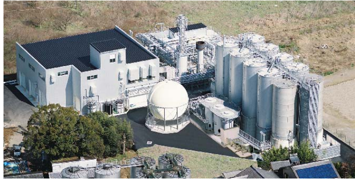
Fig. 8.2.3. Example of a large scale biomethanation plant of food waste. (Distilled spirit processing waste recycling plant of Kirishima Shuzo co. LTD.)
