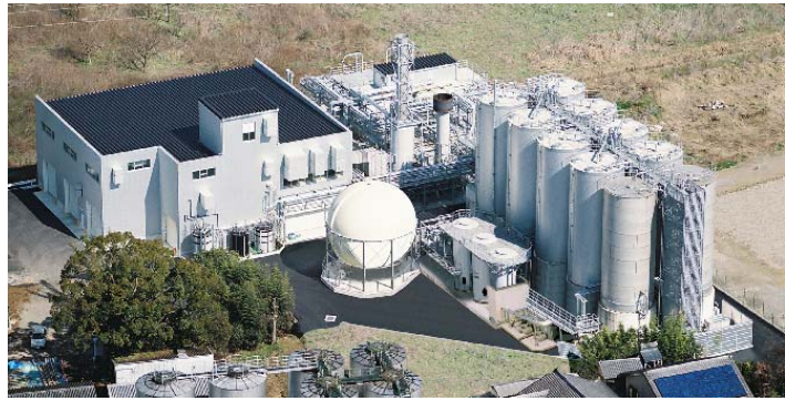
Fig. 8.2.3. Example of a large scale biomethanation plant of food waste. (Distilled spirit processing waste recycling plant of Kirishima Shuzo co. LTD.)
