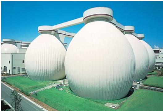
Fig. 8.2.2. Example of a large scale sewage sludge anaerobic digester. (Northern second sewage treatment plant)
